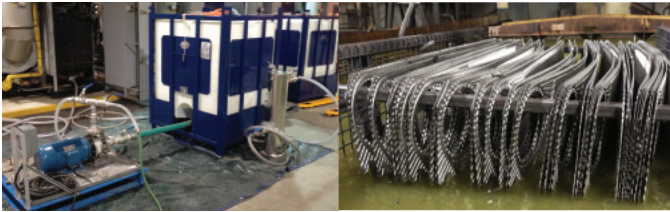
ONSITE CHEMICAL FLUSHING, HIGH PRESSURE CLEANING & OFFSITE CHEMICAL DIPPING
