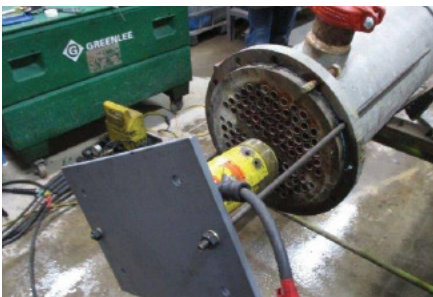
TUBE BUNDLE REMOVAL FOR REPAIR OR SERVICE
