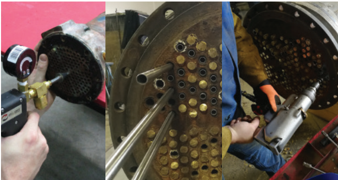
TUBE VACUUM TESTING, CLEANING, REPLACEMENT, TUBE PLUGGING, SLEEVING AND EXPANDING
